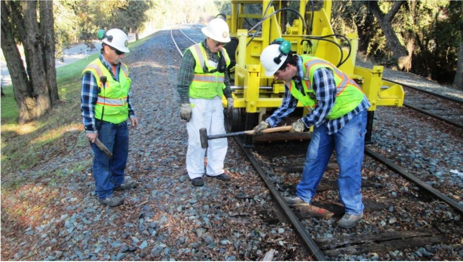
Joe and Mike H. watch Weston remove rail-anchors
