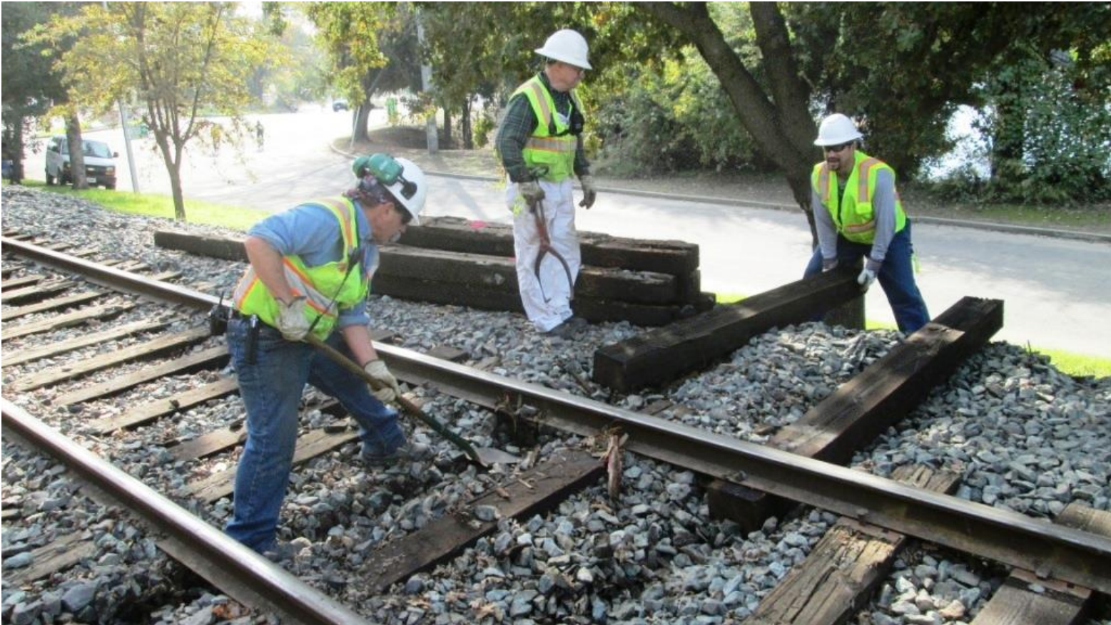
As Joe digs-out under the crib, Jose slides a tie under the base of the rail for the 125 to pull-in
