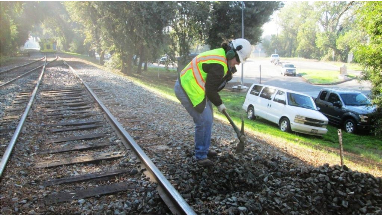
Heather digs-out a tie-crib so that the new tie can be inserted straight and level
