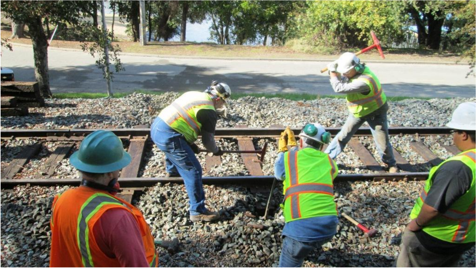
With the spikes set, Mike W. nips-up the tie as Mike F. and Steve put on a tandem spike-driving demonstration
