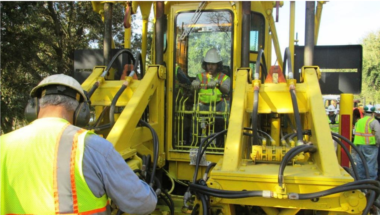
Alan guides from the ground as Matt takes a turn at operating the tamper
