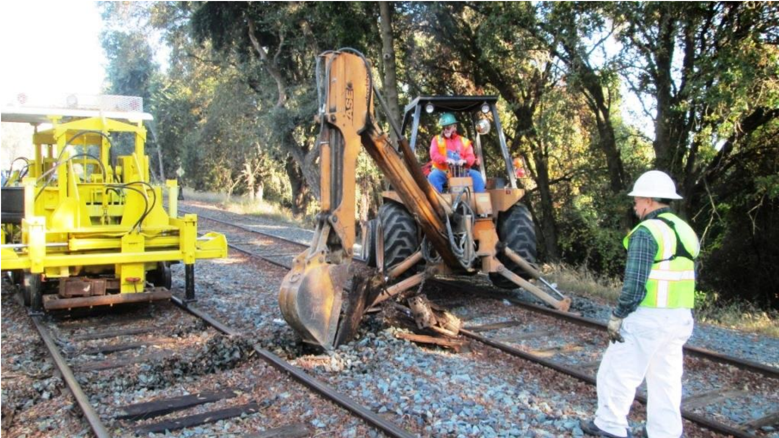
Al on the back-hoe removes a shattered tie
