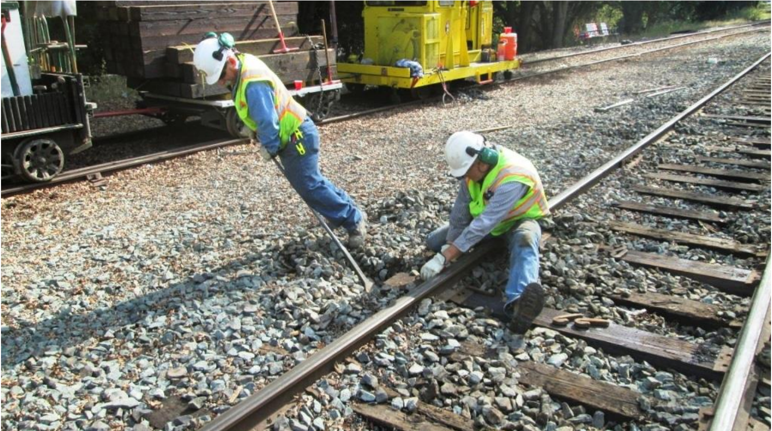
Joe puts his back into nipping-up the rail so that Steve can insert a tie-plate
