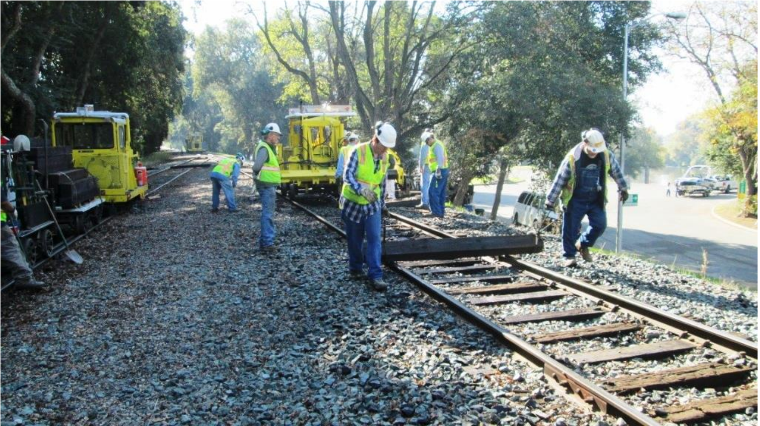
Weston and Mike F. scoot a tie along the rails to the crib where it will be inserted
