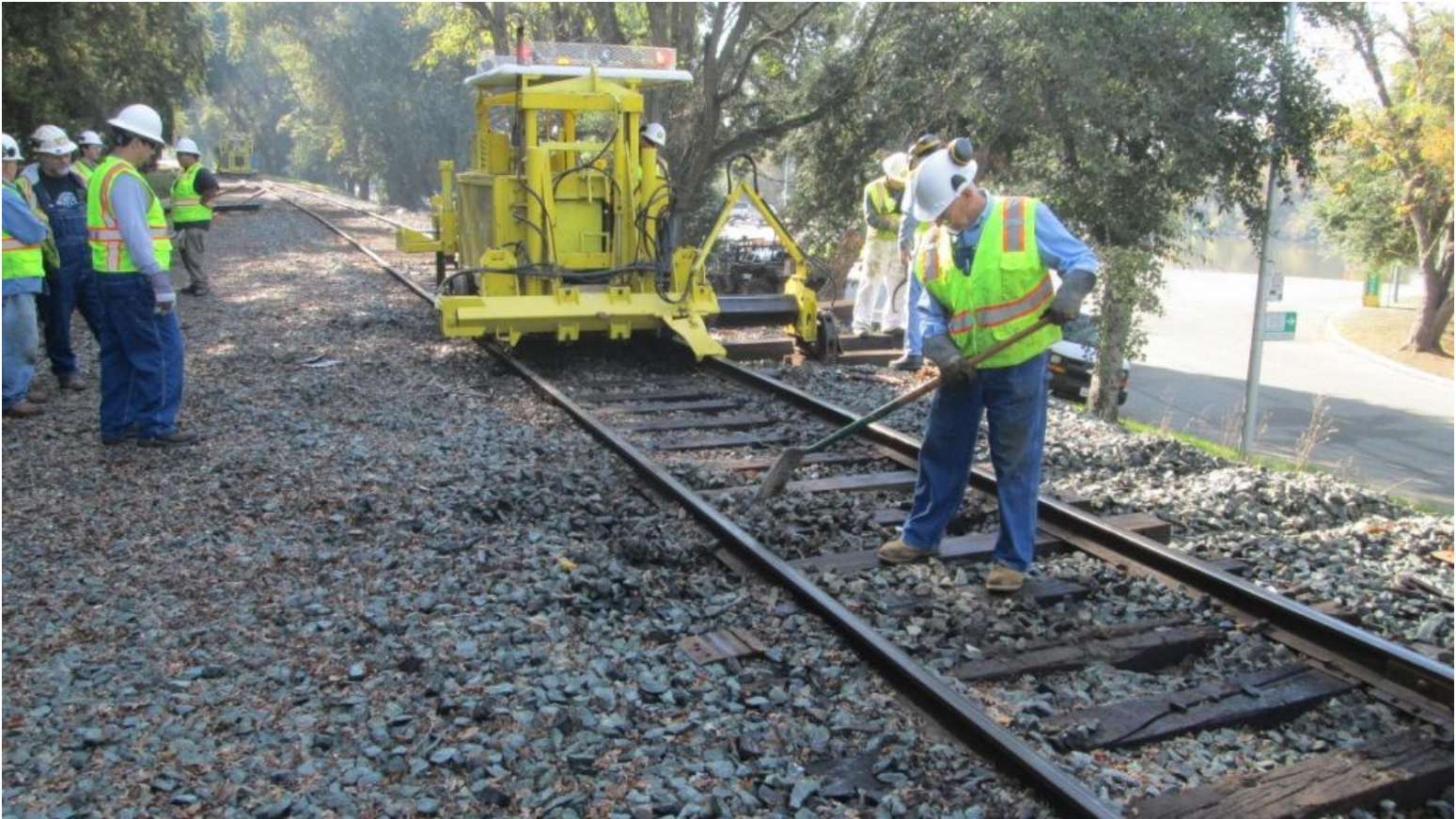
Clem fills in rock around a newly inserted tie
