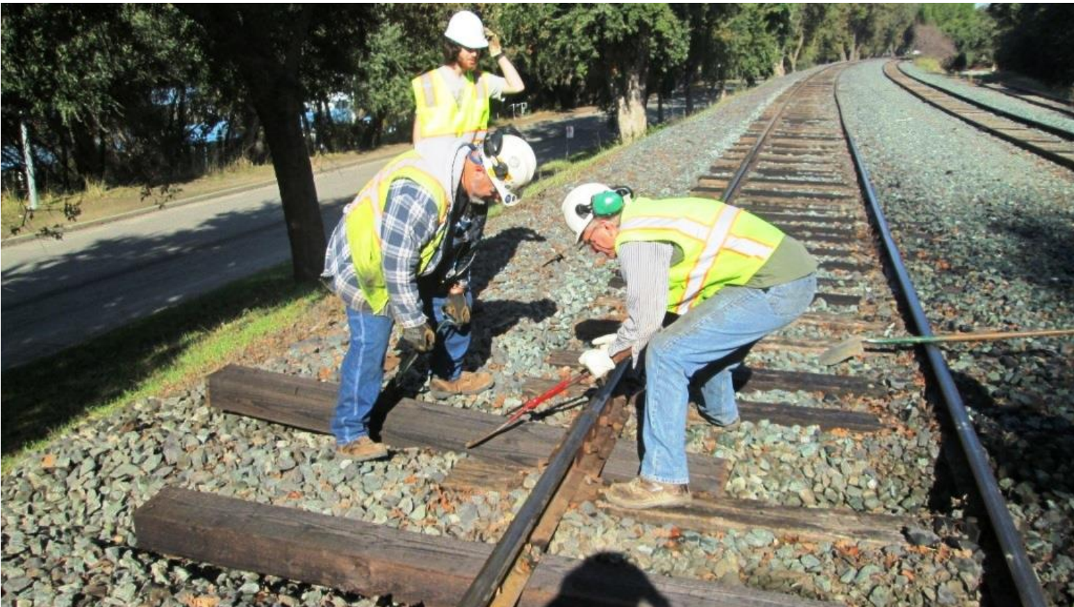
Mike F. and Steve pull a new tie under the base of the rail
