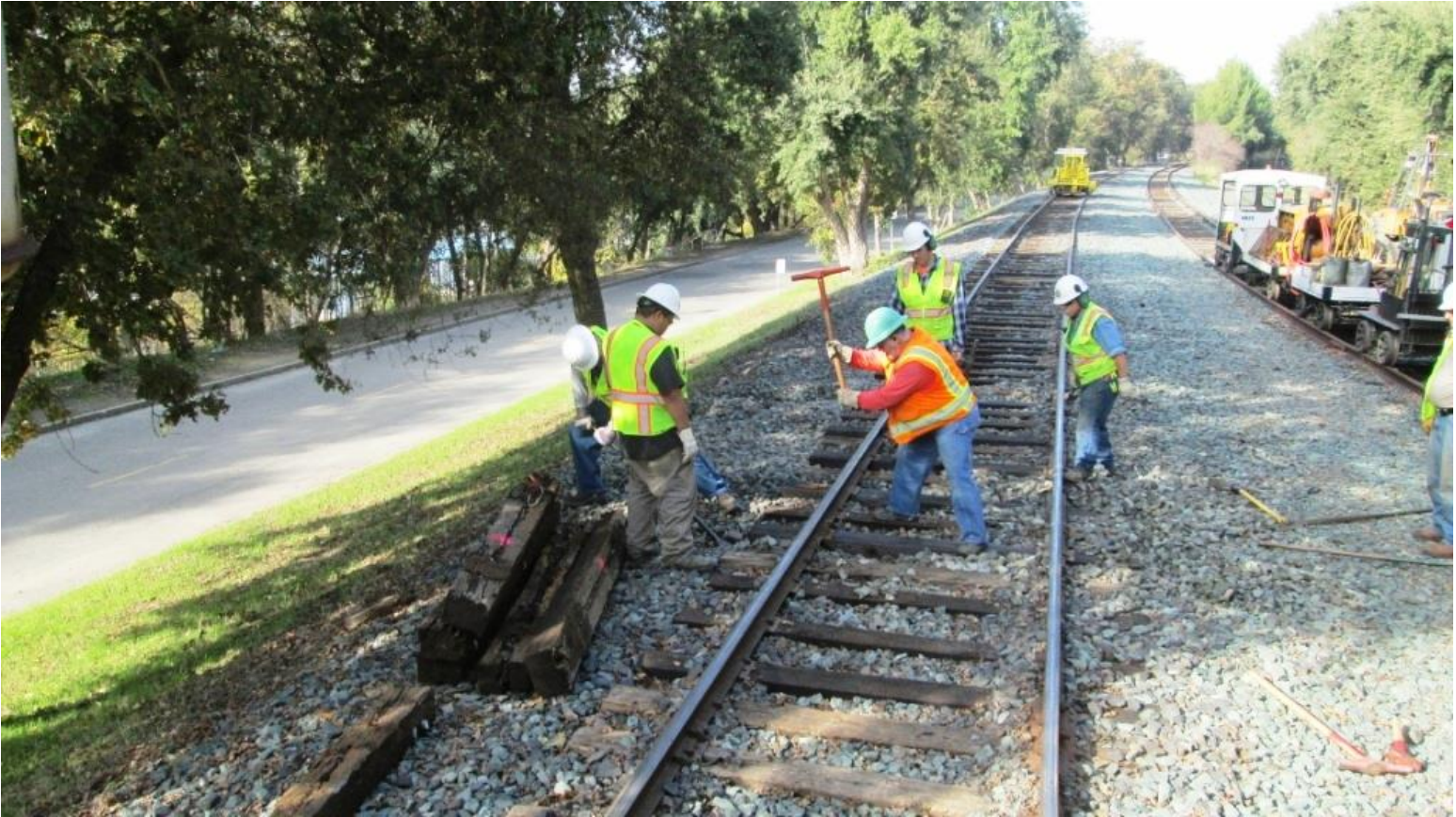
Steve nips-up the tie as Al drives a spike
