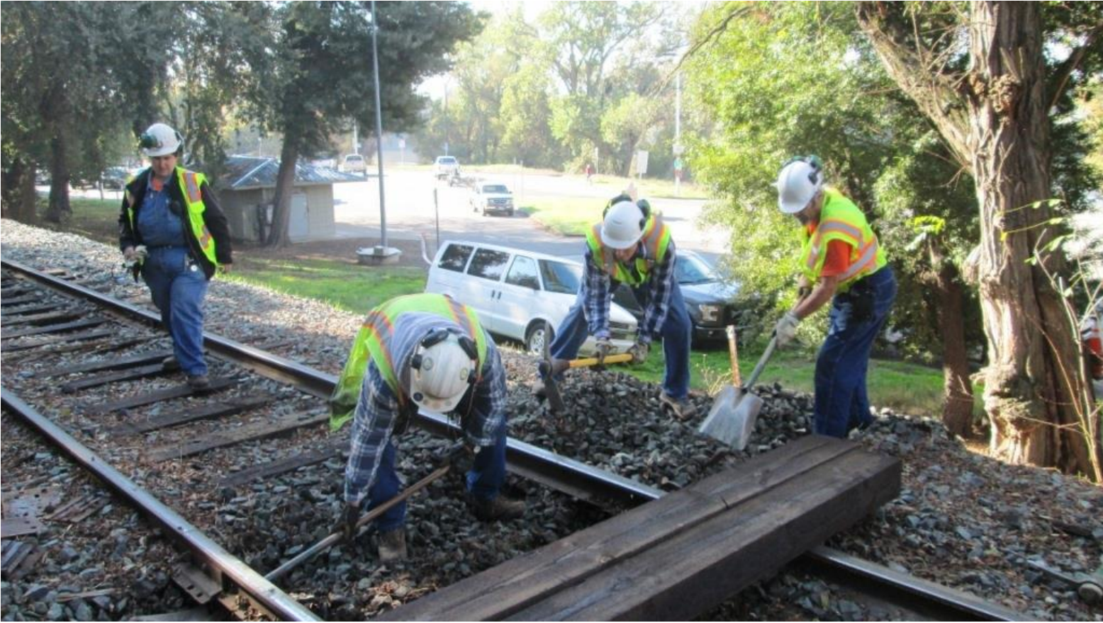
Mike F., Weston, and Ed join Heather in digging out cribs
