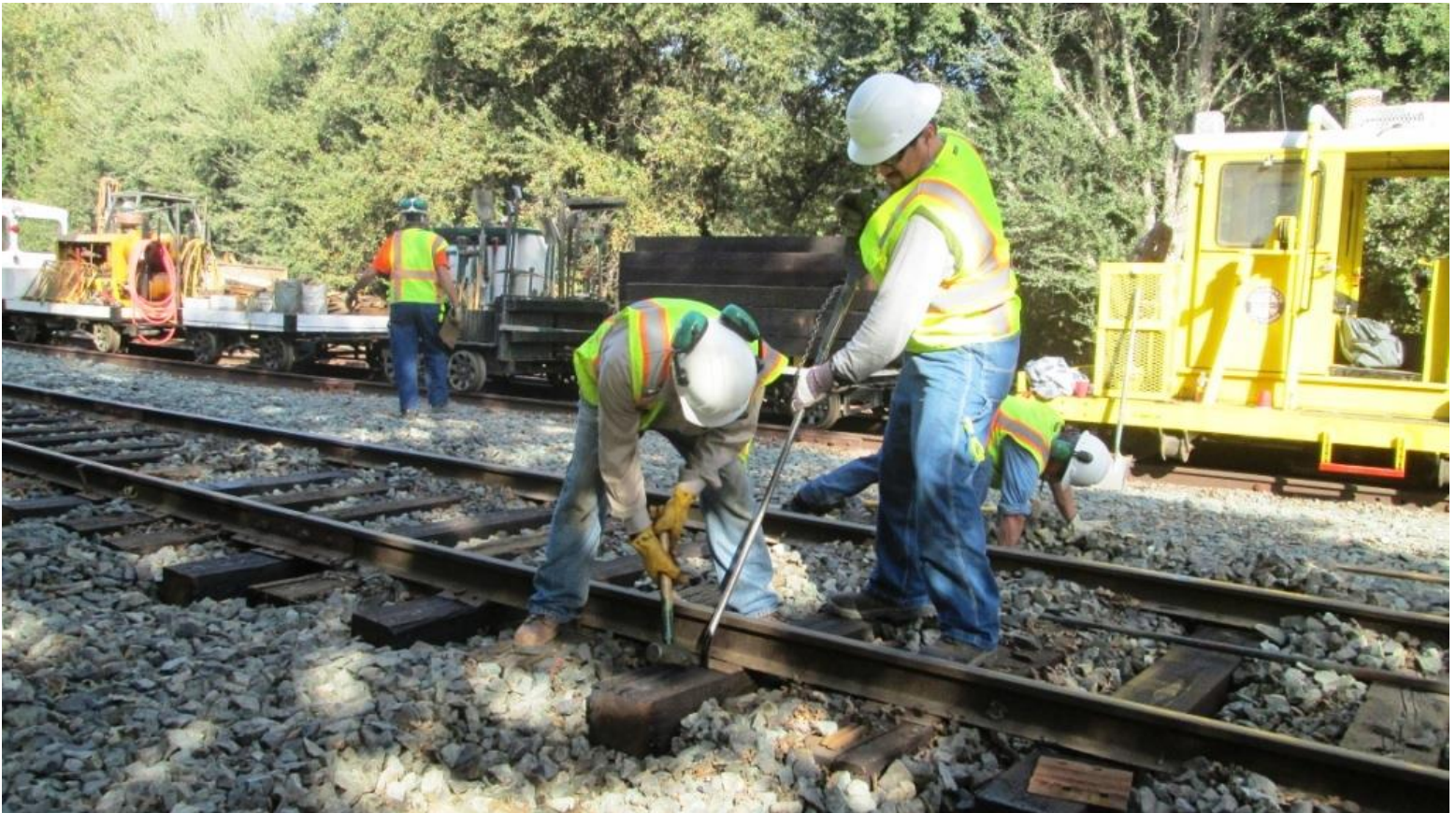
Jose places the wedge-end of the nipper-bar against the edge of a tie-plate which Steve hammers into place
