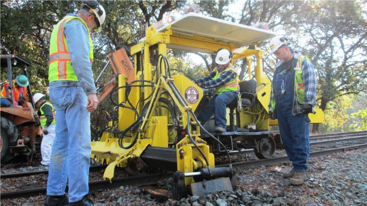
Joe on the Jackson 125 tie-exchanger removes ties
