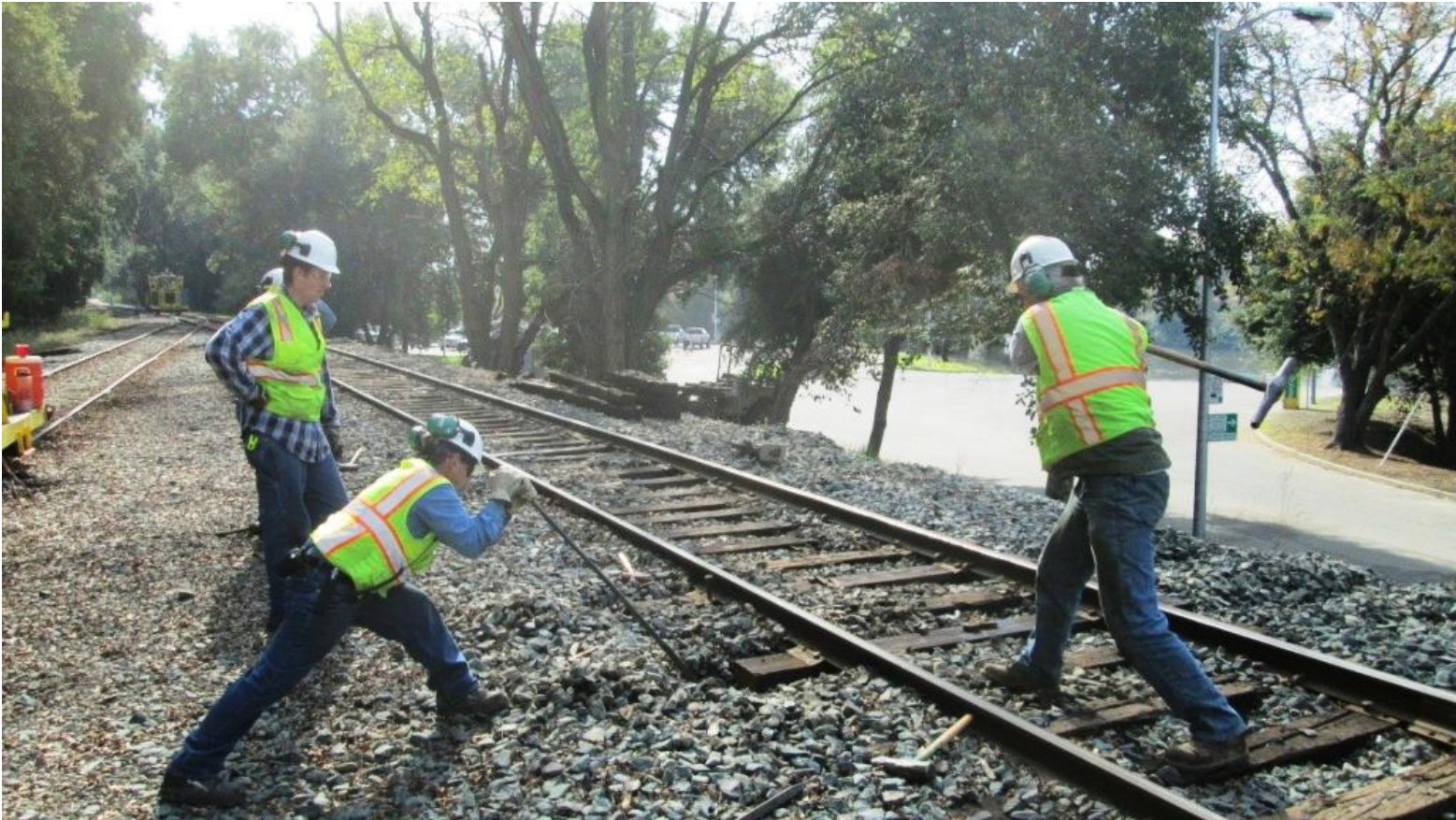
Joe nips the tie as Steve drives the spike using his world-famous as-seen-on-TV windmill spike-driving technique
