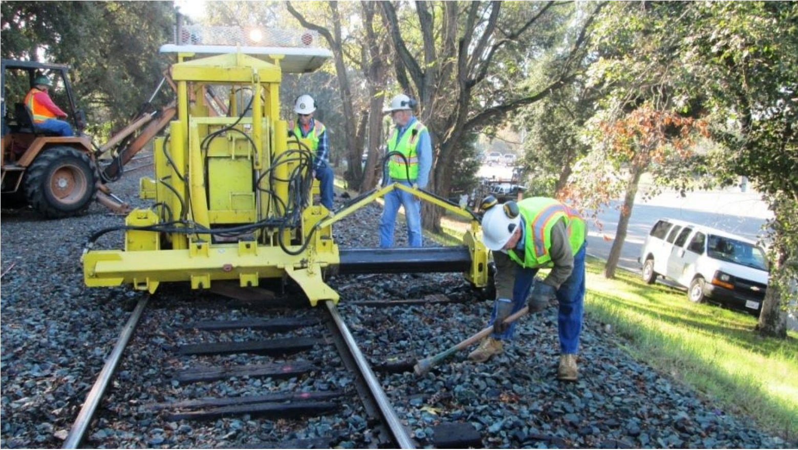
Joe on the 125 continues to remove ties as Clem works ahead to dig-out tie-ends
