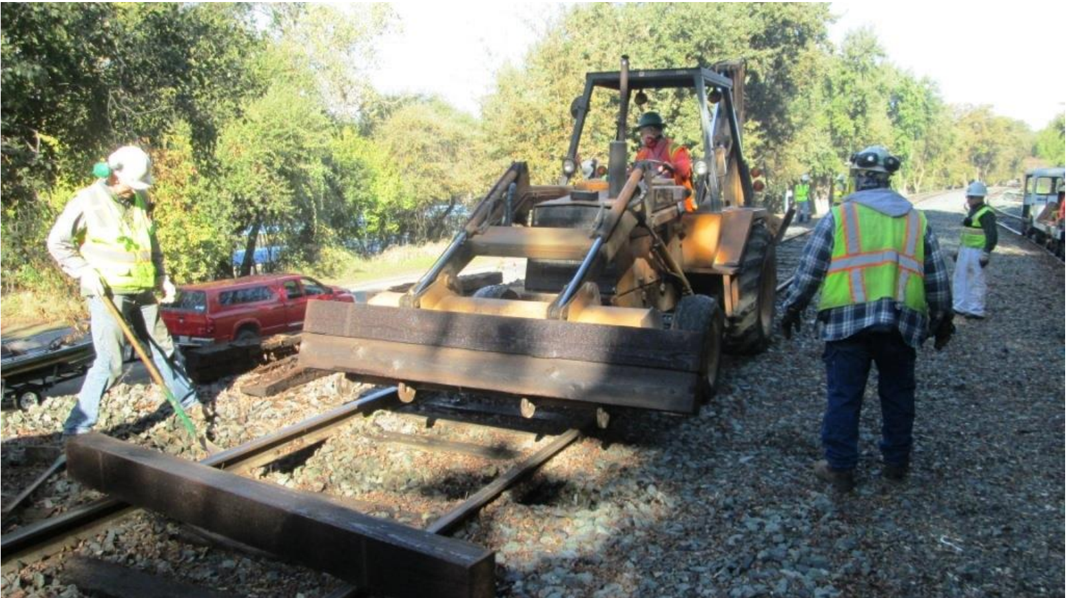
Al uses the bucket of the back-hoe to transport new ties to their new homes
